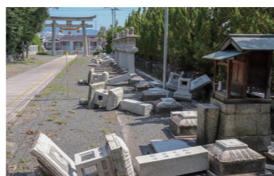
震灾中倒塌的灯笼
