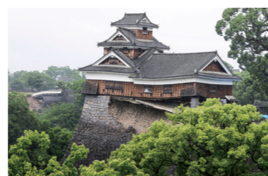
Kumamoto Castle's stone walls destroyed by the earthquake
