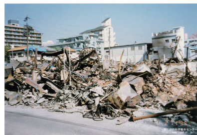
Damage to residential houses and spread of fire (1995 Great Hanshin-Awaji Earthquake)
