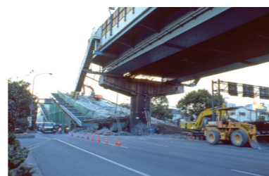
Collapsed Hanshin Expressway
