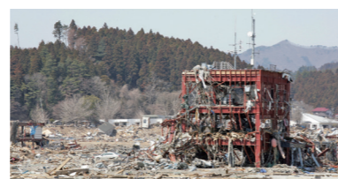
The Minami-Sanriku Disaster Prevention Office Building immediately after the earthquake
