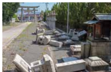
震灾中倒塌的灯笼
