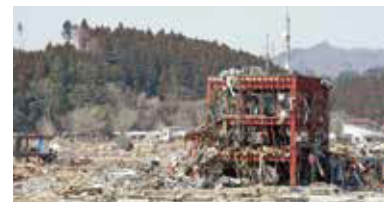
The Minami-Sanrikucho Disaster Prevention Office Building immediately after the earthquake
