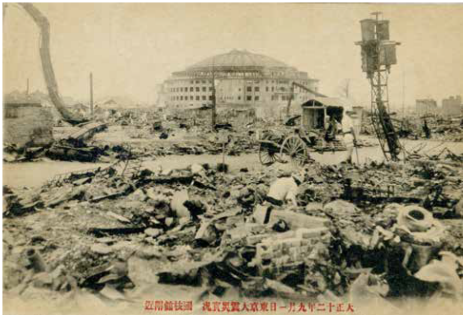
Charred ruins of the original Kokugikan building
