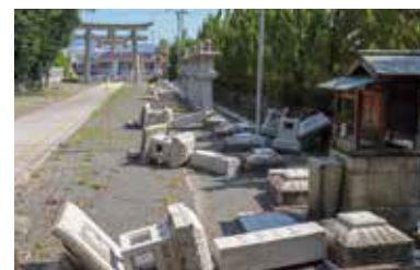
Stone lanterns toppled by the earthquake
