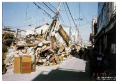
Damage to residential houses and spread of fire (1995 Great Hanshin-Awaji Earthquake)
