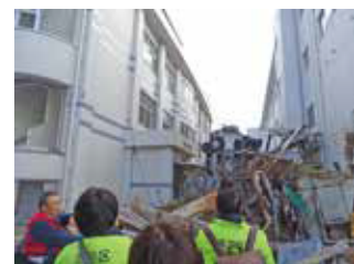
Survey of affected area
