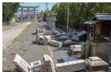
震灾中倒塌的灯笼
